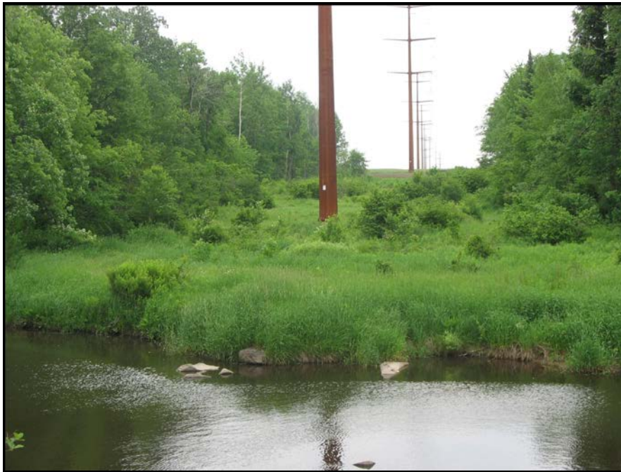
Figure 6 Restored River Bank Following Construction
