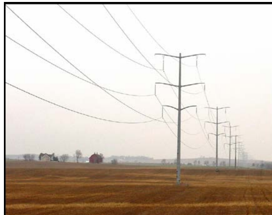
Figure 2 Typical Single-Pole, Double-Circuit Structure
