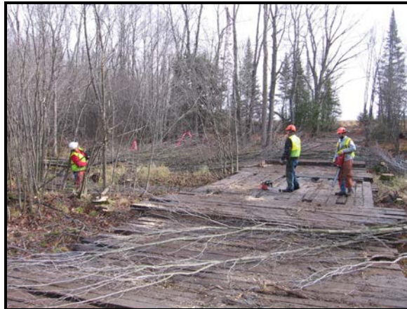
Figure 10 Hand Clearing Channel
