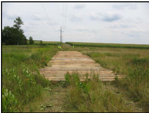
Figure 7 Mats Used in a Wet Meadow
