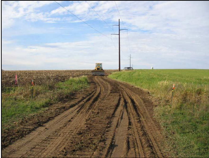
Figure 4 Smoothing Out Ruts by Backblading with a Dozer
