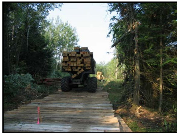
Figure 8 Mats Used in a Wooded Wetland
